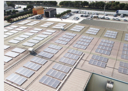
Solar panels installed at Kashima feed mill
